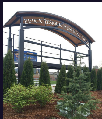
Moving Tesarik Ball Fields from its original site, along with the construction of new bleachers, dugouts, fencing and play field refurbishing, has made it the premier field for Little League.
